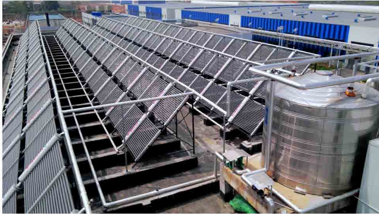
Hubei Golden Mountain Industrial Zone
